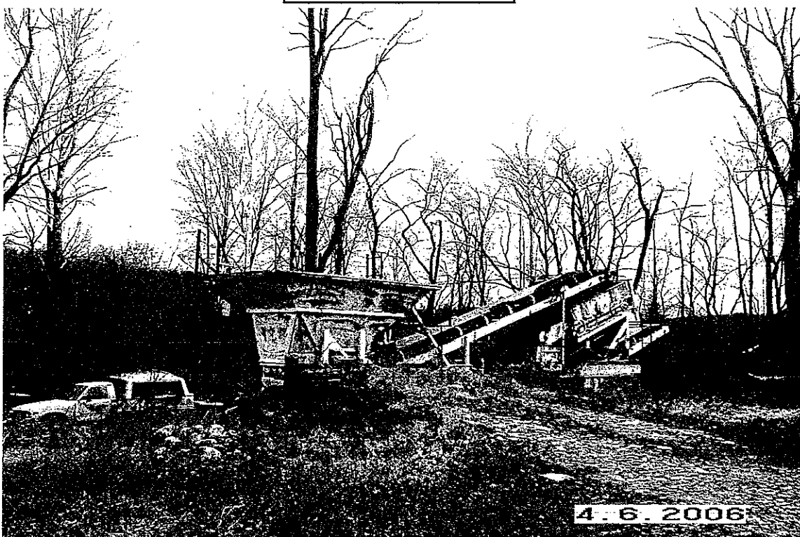
Unloading hopper and conveyer
